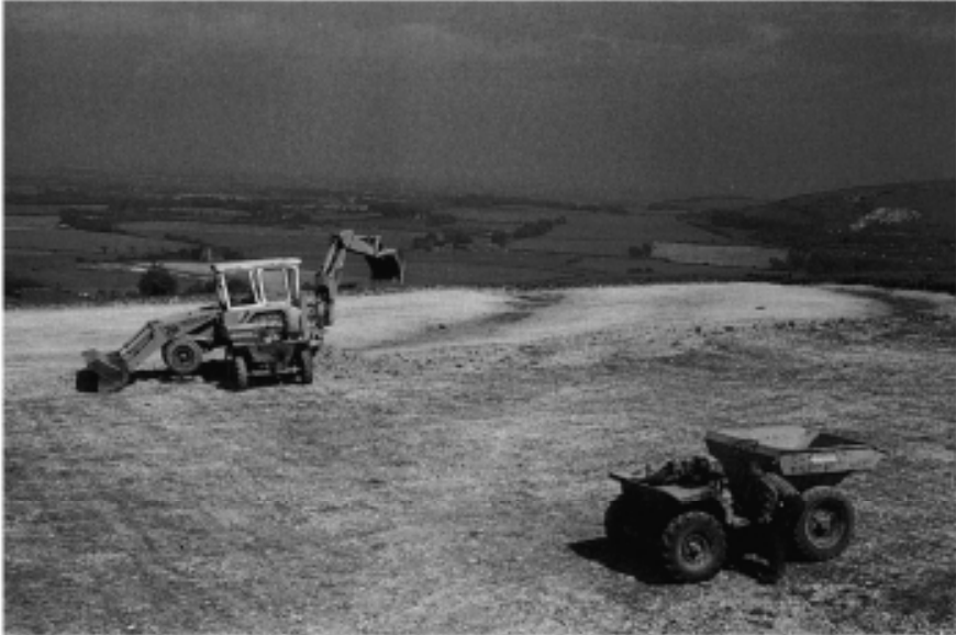
Figure 5.13 Coarse excavation: digging with a JCB 3c.
